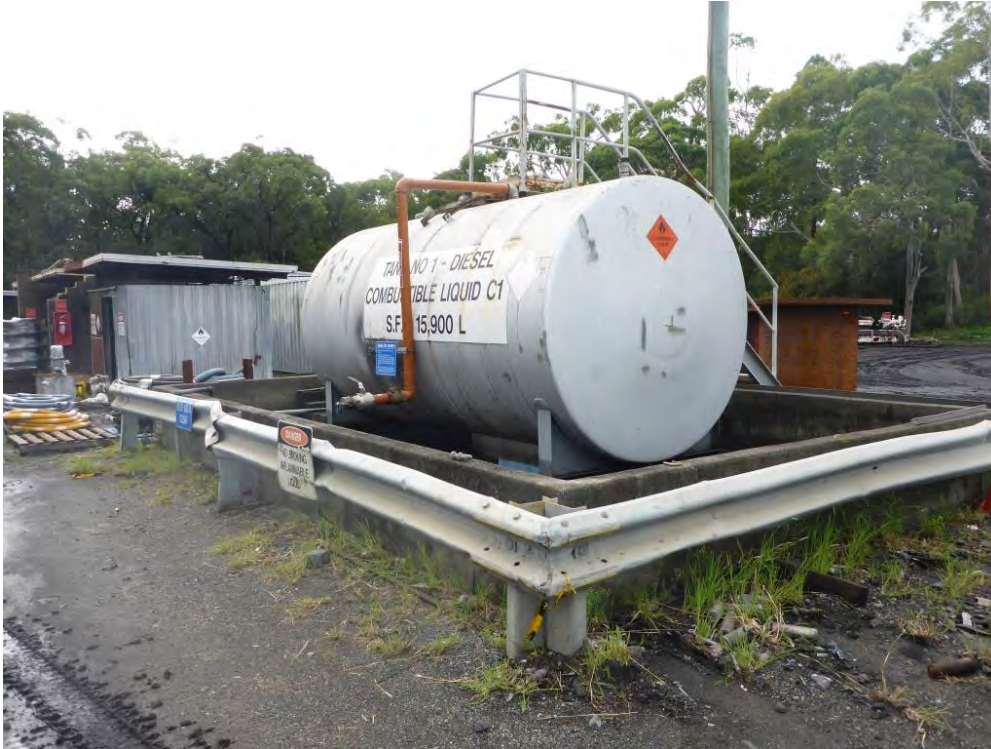
Photo 5 Diesel Tank stored within Bund
